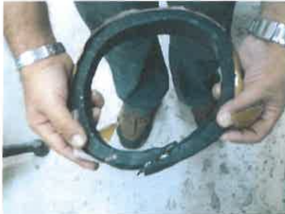
The ends of the PENEBAR SW-55 waterstop glued together with PENEBAR SW Primer
