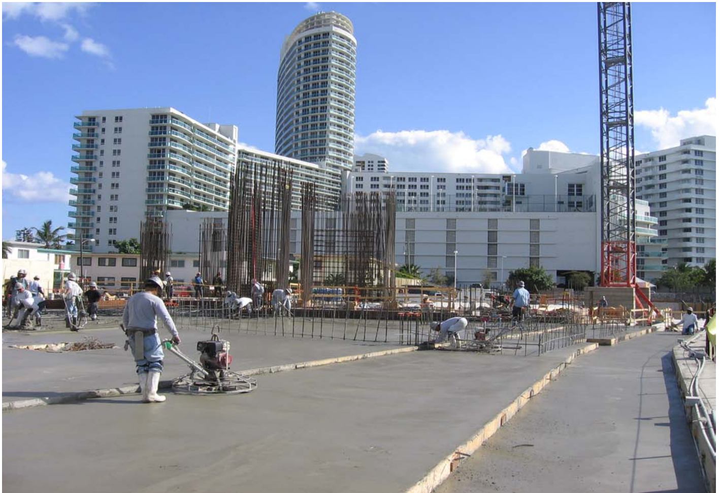
Workers applying finishing touches to the slab
