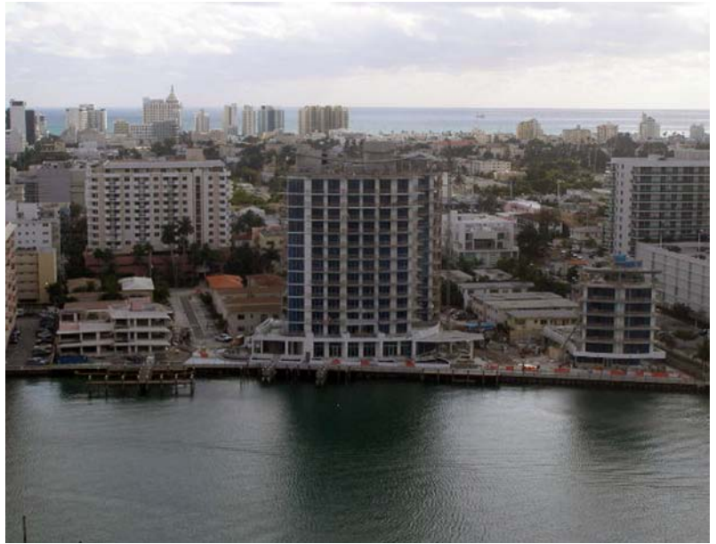
Construction in progress on the tower
