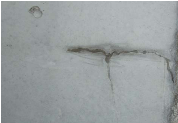
DAY 3: Crystals begin to grow filling the cracks
