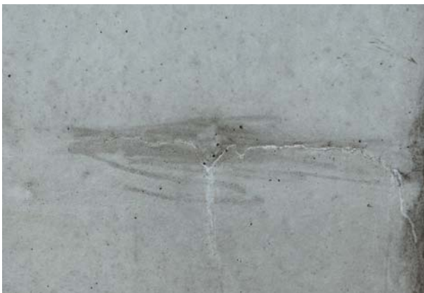
DAY 7: All cracks have self-healed and leaks completely stopped
