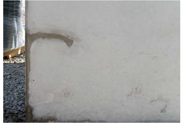
DAY 1: Leaks appear as the tank is filled
