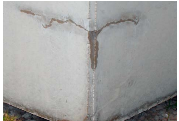
DAY 3: Crystals begin to grow filling the cracks
