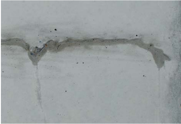
DAY 1: Leaks appear as the tank is filled
