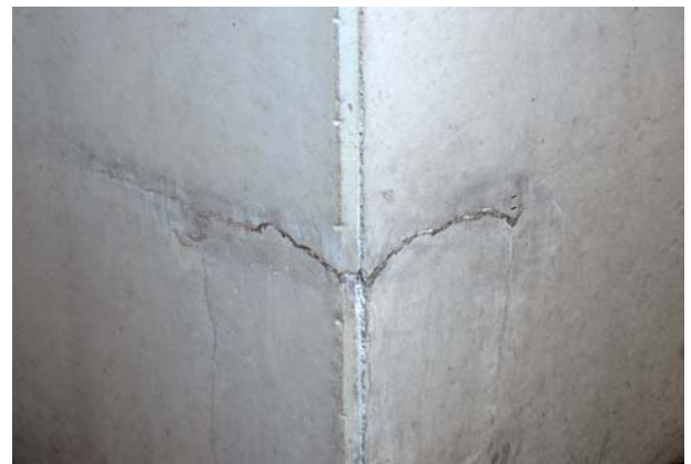
DAY 7: All cracks have self-healed and leaks completely stopped
