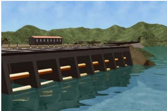
The water conductors include the power intakes, the pressure shafts and tunnels. The eight power intakes are joined together and located in an excavation next to the spillway, in the left abutment of the dam. The eight pressure shafts and tunnels convey the water from the intake to the turbines in the powerhouse.
