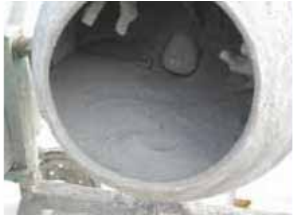
mixing Penetron with quartz sand
