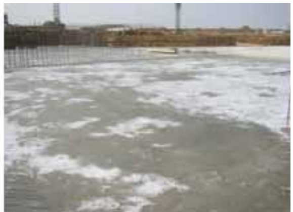
dry shake 1 day after
